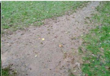
Action: Consider HIC testing impact absorbing properties to compacted; this may have an effect on the impact absorbing ensure the correct surface qualities are maintained for the equipment and replace as required
