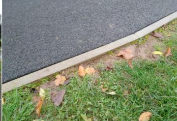
Action: Reinstate surrounding surface levels to remove the trip points
