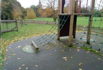
**Finding:** The rope net anchor forms a hard object within the **Action:** Monitor - No remedial work recommended impact area of the equipment in contravention of the requirements of BS EN 1176 Part 1
