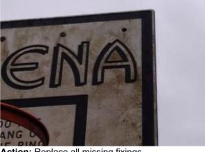
Finding: There is or are fixings missing on the backboard
