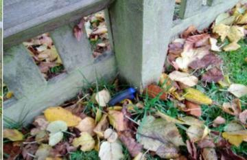
**Finding:** There are areas or parts of the timber fence posts **Action:** Replace all affected timbers on the structure that have rotted
