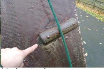
**Finding:** A number of fixing(s) have worked loose on the climbing treads
