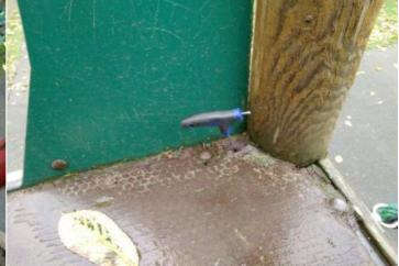
**Finding:** There are areas or parts of the slide timber platform on the structure that have rotted
