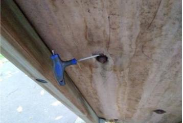
**Finding:** There are areas or parts of the timber climbing ramp the structure that have rotted
